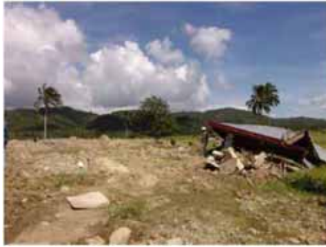
Fig.3 The roof of two story house under construction which was transported for around 200m. Within 4 persons constructing this house, 2 persons climbed the Palm tree in the left and 1 person climbed the Santol tree in the center and 1 person was killed.
