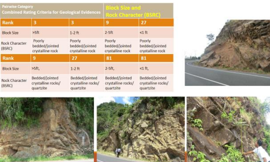
Fig 2: On site evaluation of Block size and Rock Character
